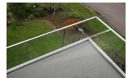
1.2m high strengthened glass balustrade
