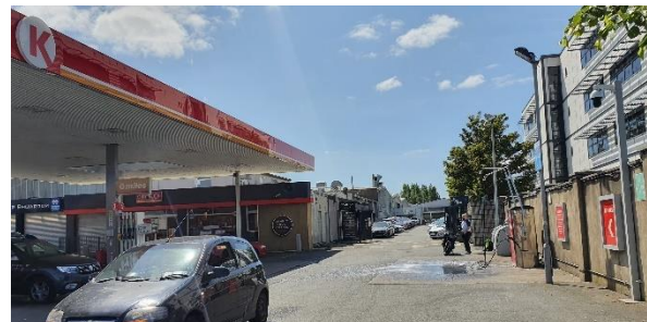
3. View along the north-eastern boundary of the site
